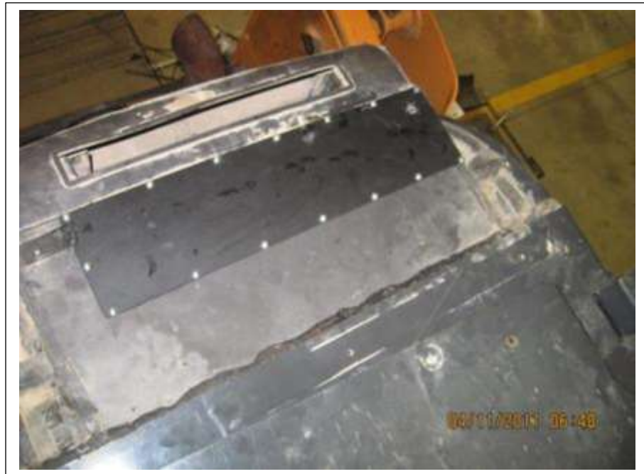
Cover fastened in place
