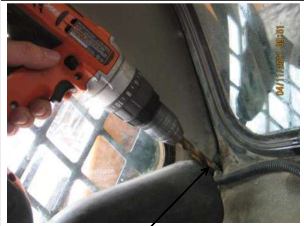
Drill hole to send drain tubes through
